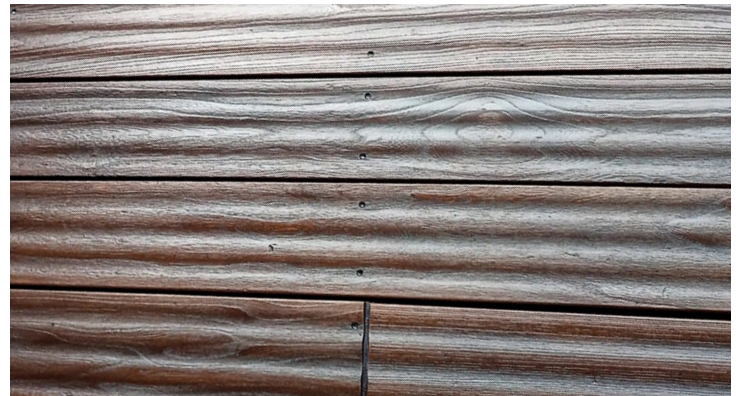
Renovated deck made from thermally treated ash after finishing with DeckFinish Color in dark brown.
